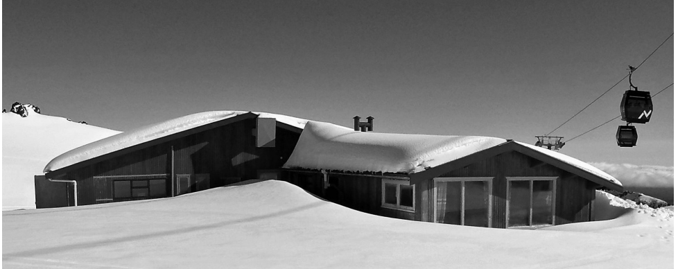
RSC Hut and the Sky Waka gondola. Photo: Peter Otway.
